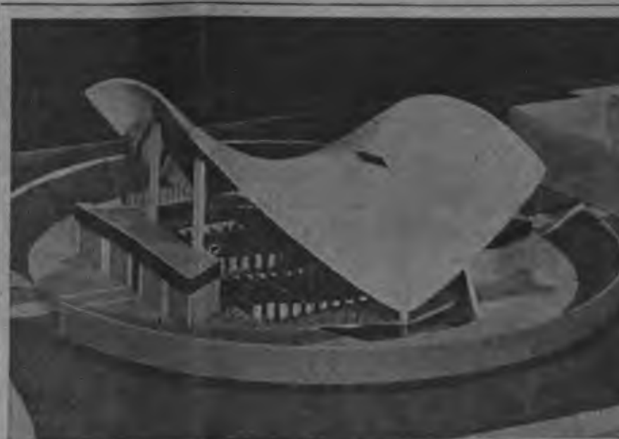
This is a preliminary model of the proposed St. John's Church, Ermine Estate, Lincoln, designed by Mr. Sam Scorer, the Lincoln architect. The all-concrete roof will have no internal pillars. The external struts shown in the picture here will be filled in with bricks and glass. (See Page 5).
